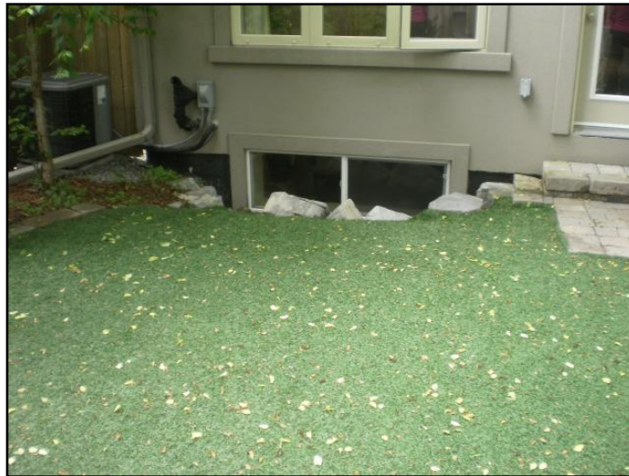
17. Improper slope
