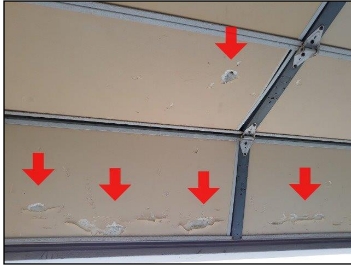
18. Damage- garage vehicle door
