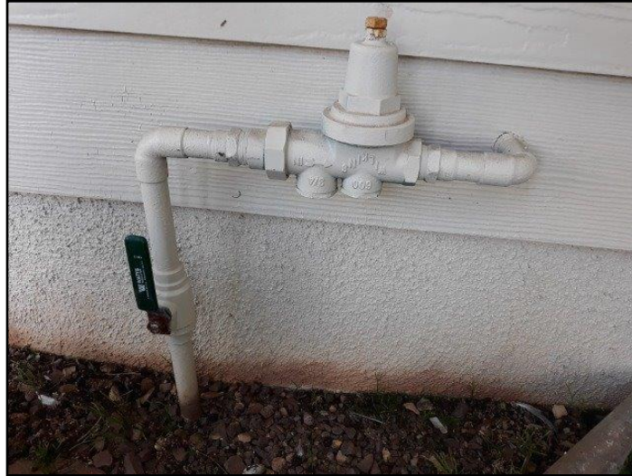
55. Water shut-off and pressure regulator
