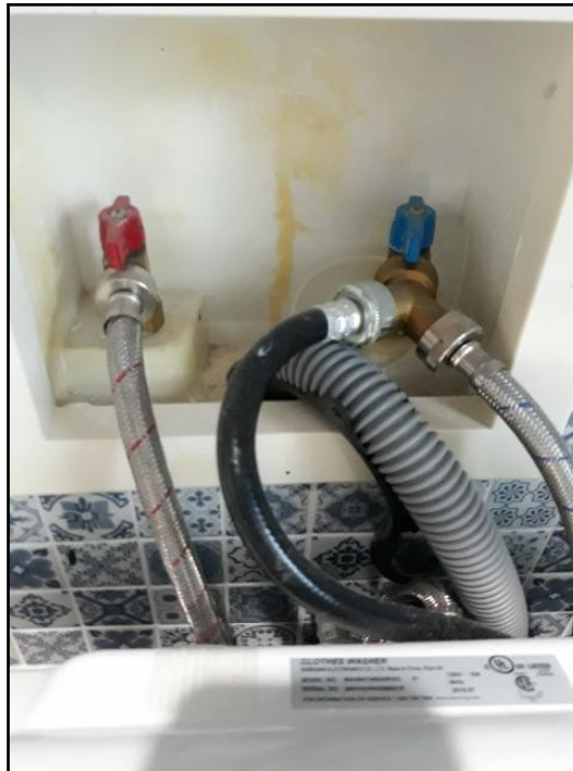
86. Water supply and standpipe
