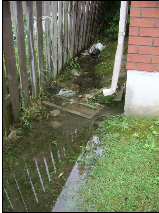
14. Downspouts end too close to building
