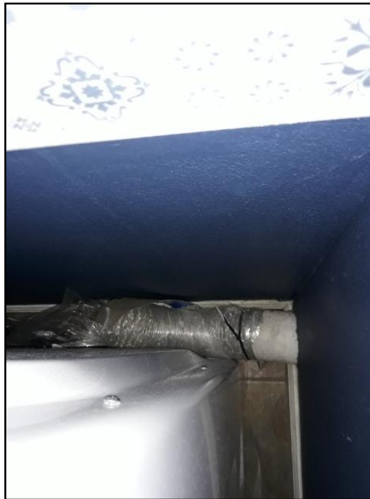
88. Clothes dryer vented to exterior
