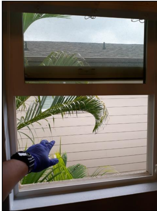
90. Missing window screen- bathroom
